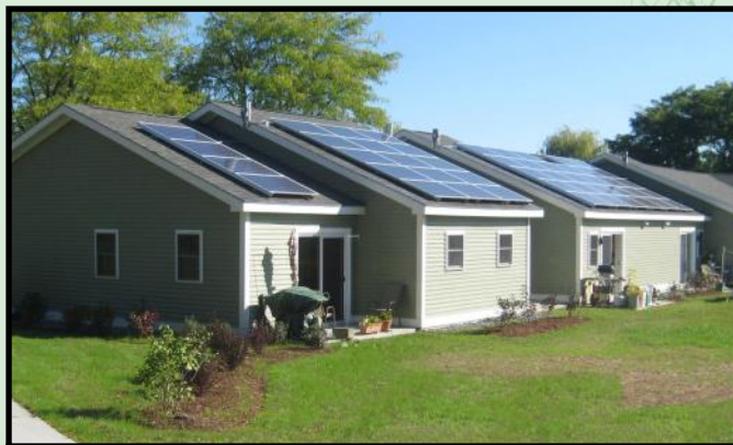
New solar hot water/photovoltaic system at recently renovated Valley View II Apartments in Vergennes (picture: NBF Architects )
